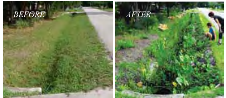
Bioswale before and after completion.
